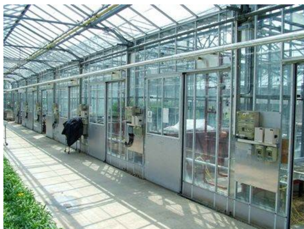
Figure 1: Temperature-controlled glasshouse compartments.
